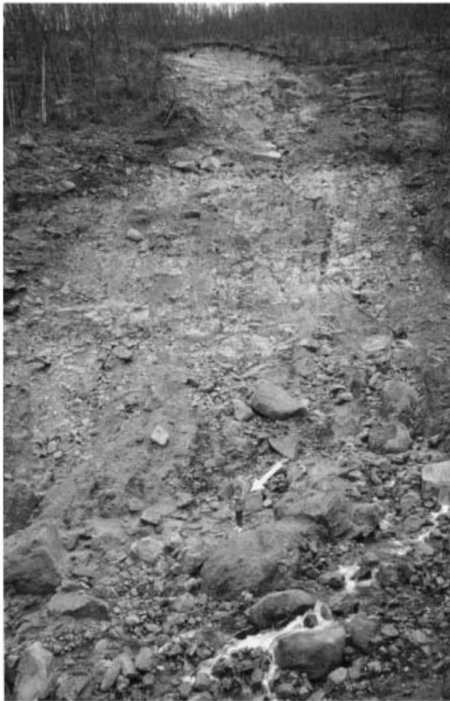
Figure 4. (A) Surface rupture of the Jubaguerra debris slide, displacing regolith materials (to see the scale, note the person pointed by an arrow). (B) The first sequence of debris flood deposit along the Jubaguerra stream. It took place after the first sequence of riverbank erosion and just beyond the first small waterfall (it can be seen on the right upper corner of the figure).
